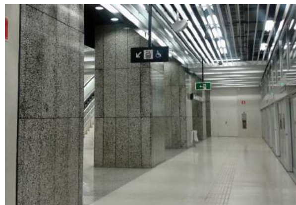
Metro station L9 Parc Nou, example of the new metro stations of L9 that connects Barcelona with the airport
