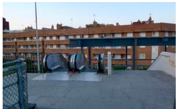
Photos that illustrate more details of the bridge that connects Santa Eulàlia with Collblanc
